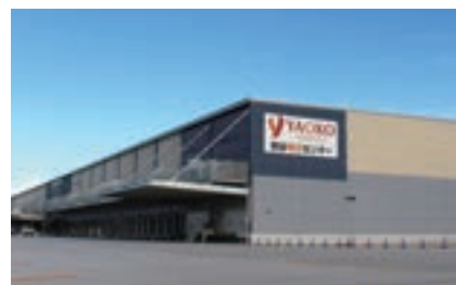
Kumagaya Distribution Center
