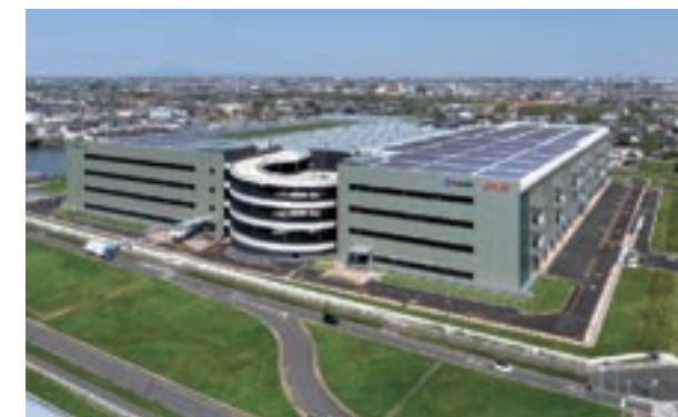
Soka Distribution Center
